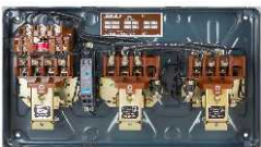
Interior View of MK2 FASD
