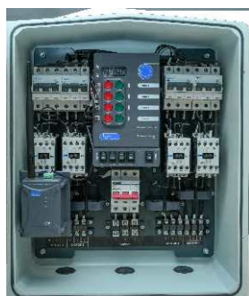
Interior View of xMU-GiA
